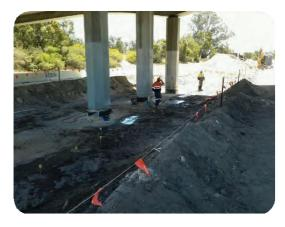
Permeation grouting can be used to solidify and to create a 'stable mass' from the existing unstable sands and other non-cohesive soils at depths.
