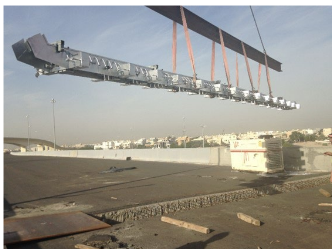
→ EJ safely lifted with crane and inserted in position
