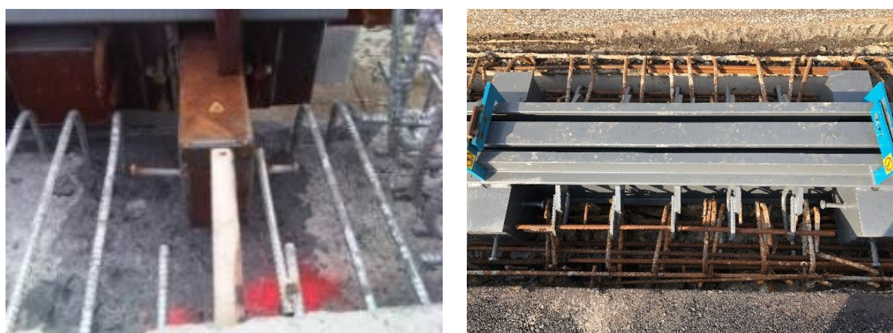
→ New rebar welded to the existing one as a temporary support of one side of the EJ.
