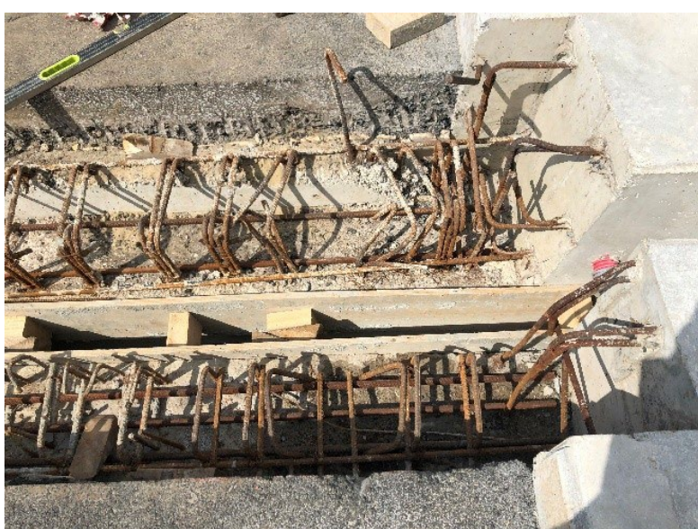
→ Adjustment of the rebar to host the joint box as needed.
