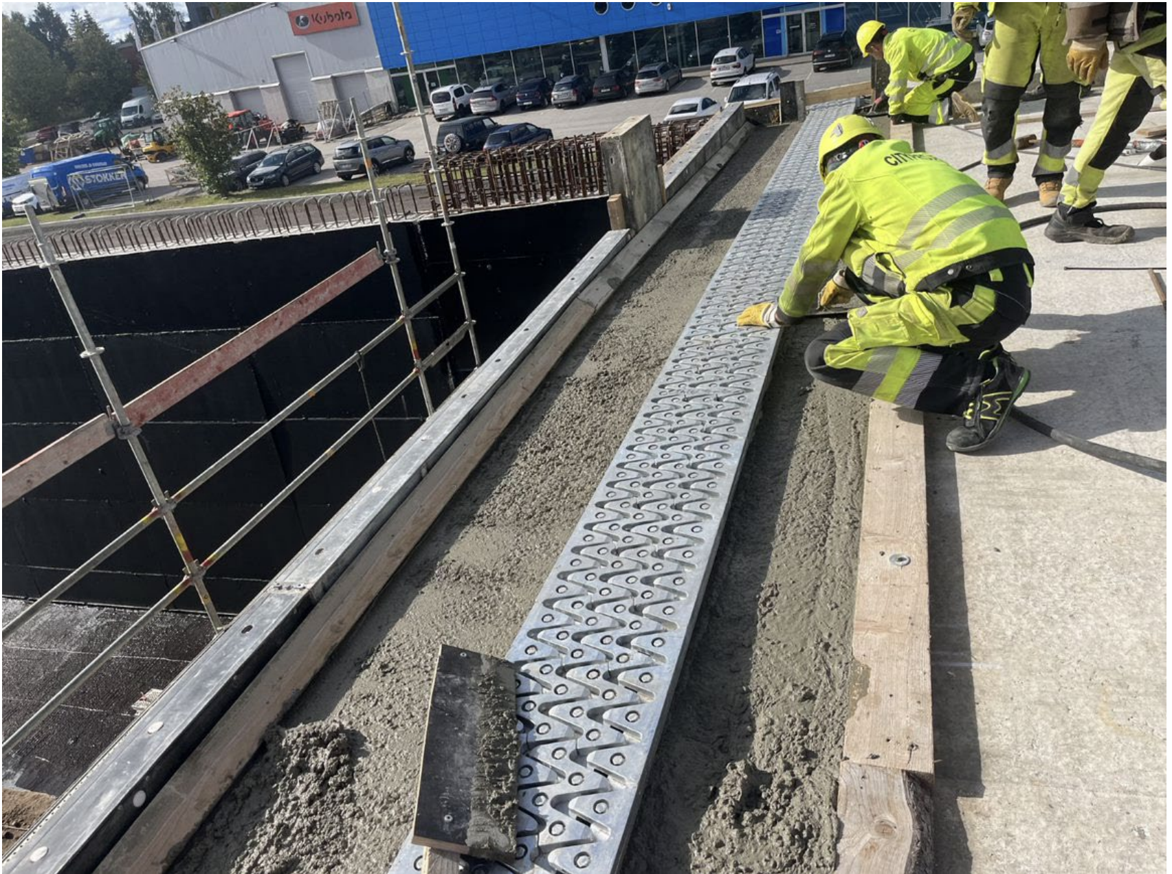
MEJ during concreting
