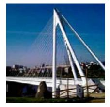
Basic stay is fully sealed to avoid the entrance of water inside and comprises at least 4 protective barriers to the steel of the strands at any point, this warrants the maximum durability of the tensile element against corrosion.
